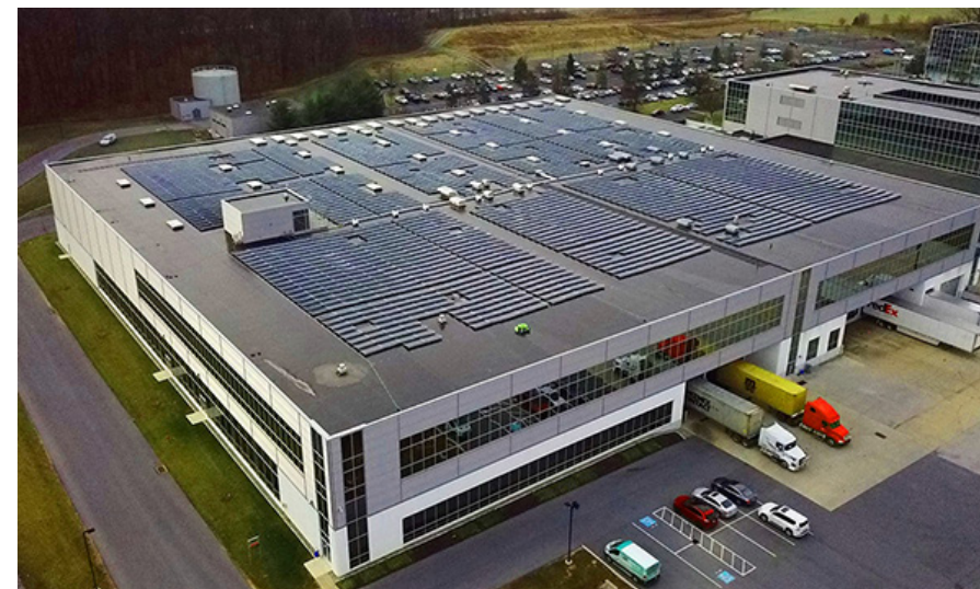
Figure 1: Rooftop PV generation was a key factor enabling this Phoenix Contact facility to achieve LEED Silver and ZEB certifications. (Image source: Phoenix Contact)
